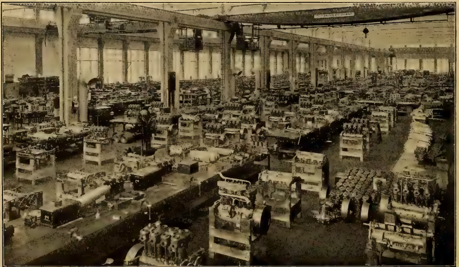
Another view of a great assembling department.
